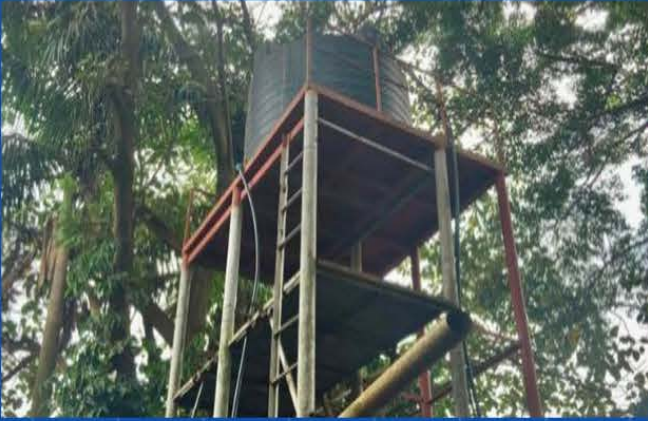
Relocation and Installation of the Water Tank
